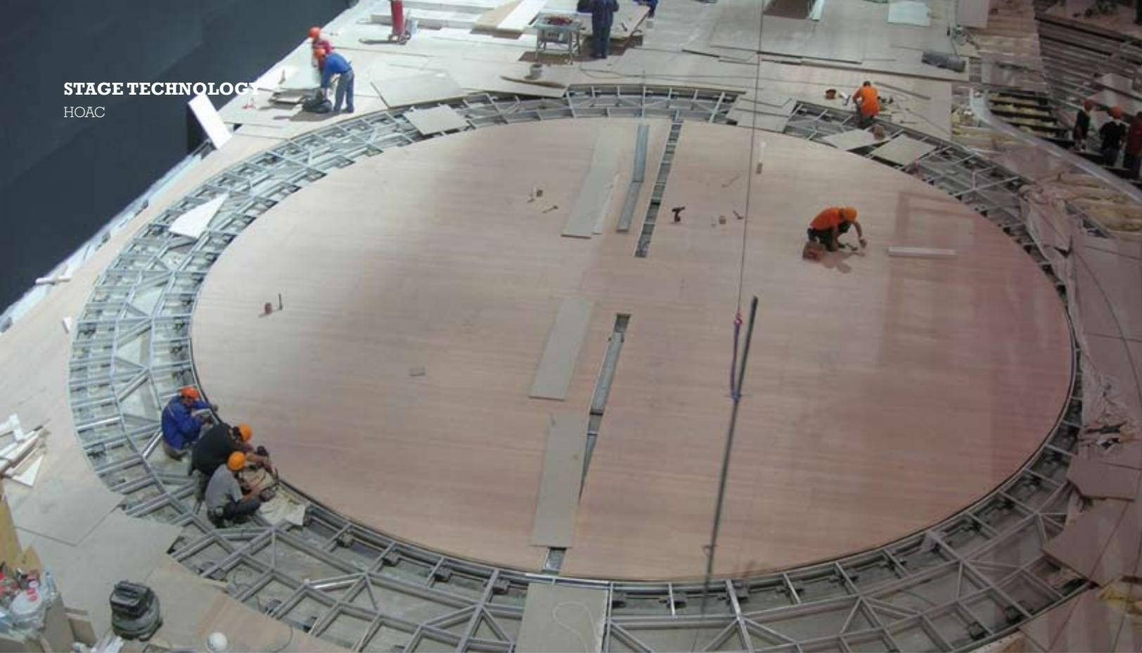
**Above: Both parts of the revolving stage are integrated into the main stage**
